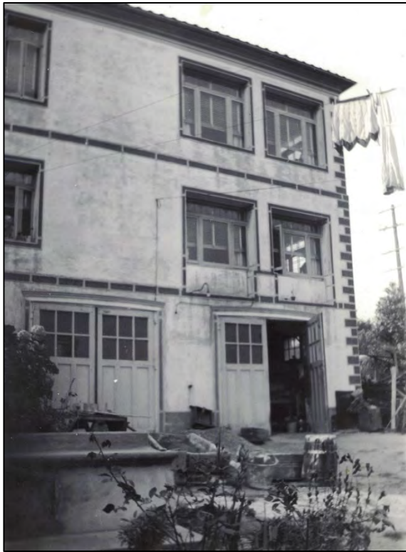
East (rear) facade
