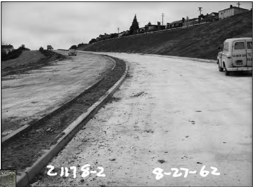
Fauntleroy Ave widening completed 1962
