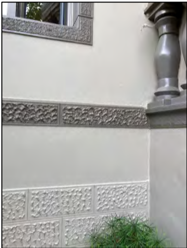
Stucco details at West (front) facade
