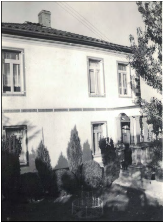
South (side) facade
