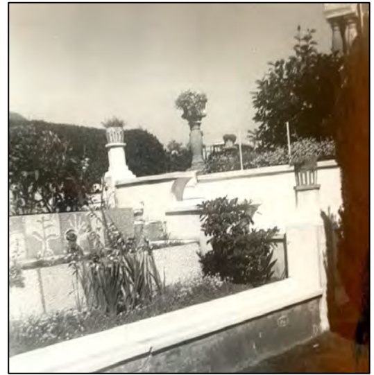
Steps at SW corner of house 1966 (partly intact)
