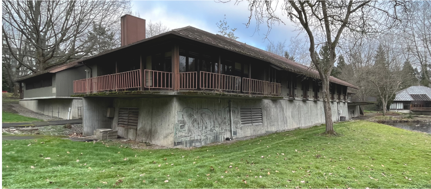
BUILDING D SOUTHWEST CORNER - EXISTING CONDITION
