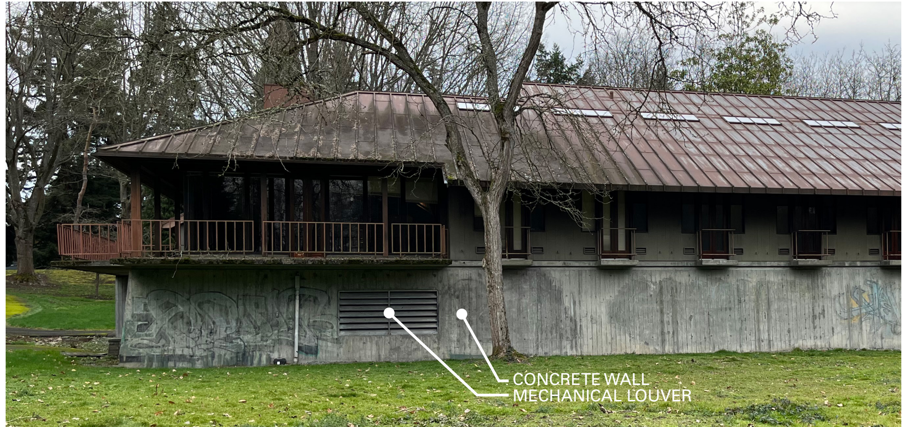
BUILDING D SOUTHWEST CORNER - SOUTH FACADE
