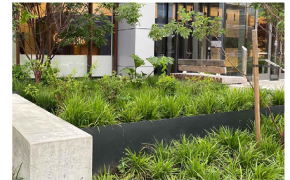
7 RAINGARDEN MANAGE SITE STORMWATER. WATER-ACCEPTING STRUCTURED LANDSCAPE HOSTING LAYERED, LOW MAINTANCE PLANTING.
