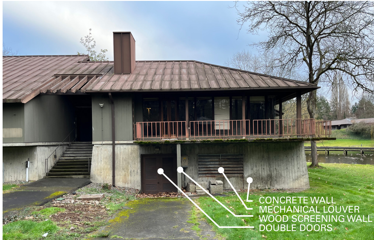
BUILDING D SOUTHWEST CORNER - WEST FACADE
