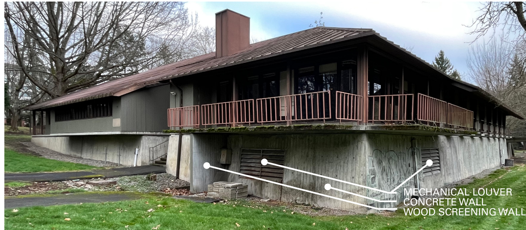
BUILDING D SOUTHWEST CORNER
