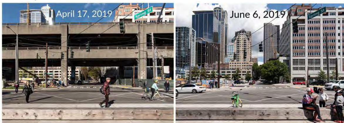
Figure 11 Removal of the Viaduct ( Puget Sound Business Journal / WSDOT )
