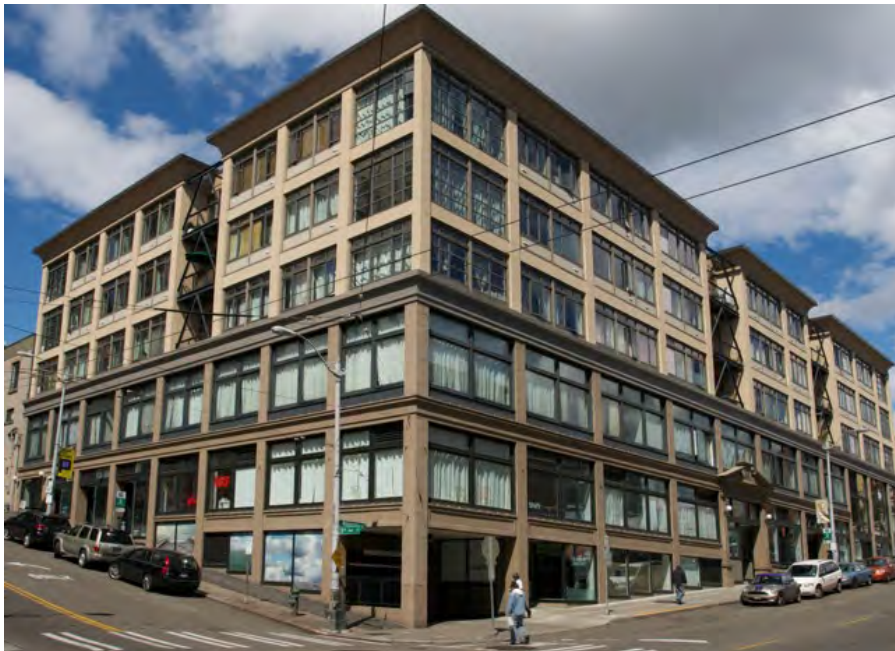
Present-day building with 6 stories of housing for artists and their families, gallery space, and studios. Image source: Art&Seek, 2014.
