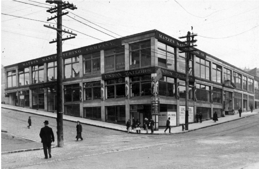
Tashiro-Kaplan building in early 1900s Image source: Artspace, 2024.
